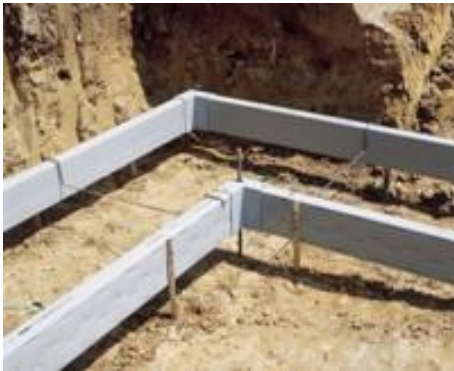
Figure 2. “Form-A-Drain” corner assembly
