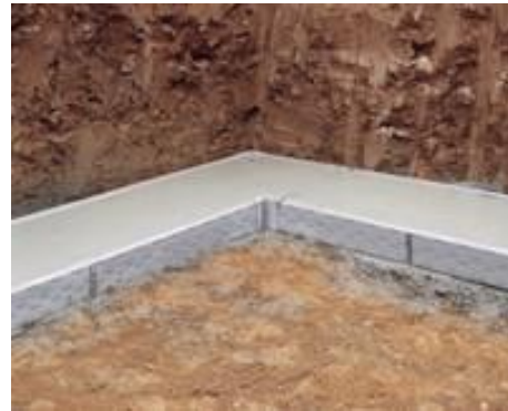
Figure 3. “Form-A-Drain” corner assembly after concrete placement
